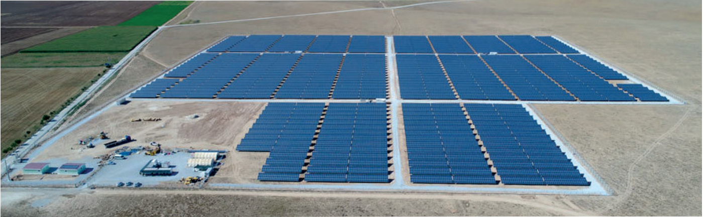
8,6 MW Konya 1 Energy Plant
