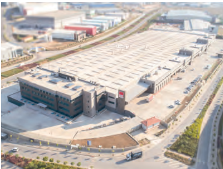
Plant 4 Busbar Factory Kocaeli / TURKEY
