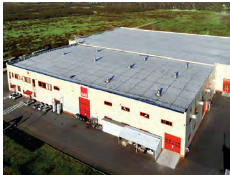
Plant 5 Busbar & Lighting Factory Aleksandrov / RUSSIA
