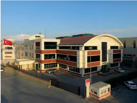
EAE Headquarters & Plant 1 Busbar Factory Istanbul / TURKEY
